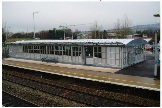
Project Name:Cwmbran Railway StationProduct:Modular Automated Ticket OfficeClient(s):Alun Griffiths ContractorsScope of Project:The design, manufacture and installation of fully fitted<br/>automated ticket office, 18m x 6m with full length platform<br/>canopies, heating, paragon seating, public DDA compliant<br/>toilets, swing doors, staff room area with ticket office, small<br/>kitchen, washroom area, store rooms and retail unit.
