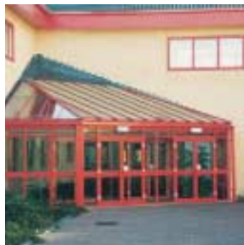
Monopitch roof with gable
