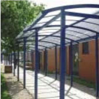
Open sided walkway
