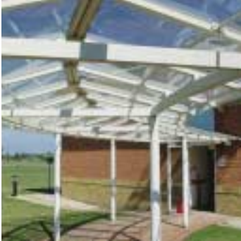
Curved roof only walkway
