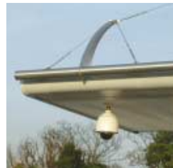
Cantilever canopy at Twickenham Station
