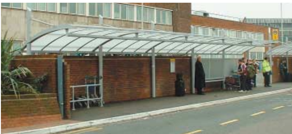
Cantilever walkway with bespoke lighting to the front
