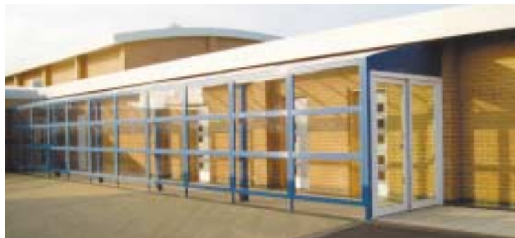
Monopitch with external glazing & infill panels
