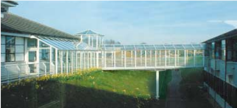
Elevated enclosed walkway
