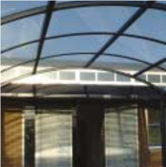
5m span low vault roof
