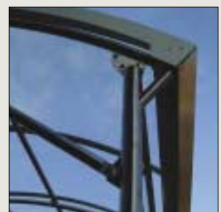
Roof frame connections
