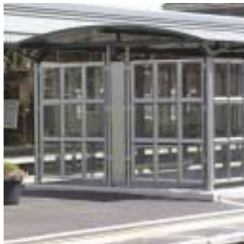
4m span with glazing
