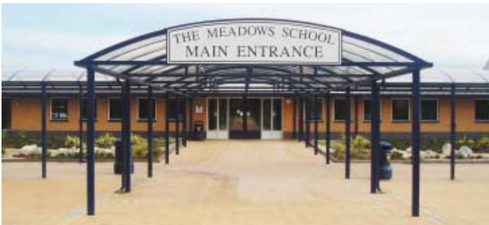
5m span low vault
