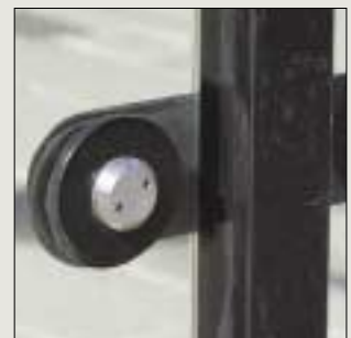
Tab fixed glass with pignose fixings
